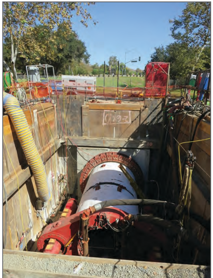
On October 3, 2012, the Santa Ana River Interceptor Mainline and Metering Station project site received a Micro Tunnel Boring Machine all the way from Oregon, shown here inside the tunneling shaft.
