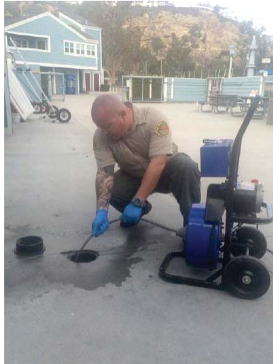
Ramiro's maintenance duties include snaking drains to make sure they are clear.
