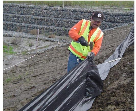
OCWR staff, Irineo Rios installs a silt fence that will slow the flow of runoff and collect the silt on slopes.
